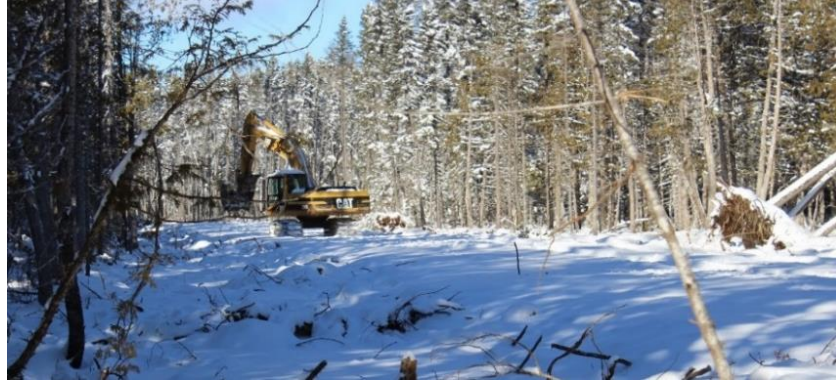
Figure 2. Winter roads constructed by a loader for transporting forest products in Maine. Winter roads are comparatively cost efficient in construction and maintenance compared to paved forest roads.
