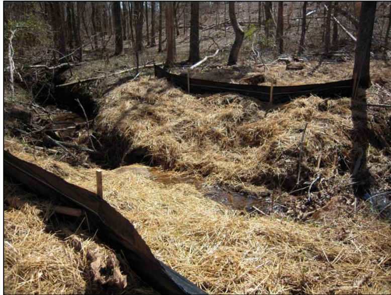
Figure 5. Representative stream crossing approach that was closed with mulch + silt fence treatment.
