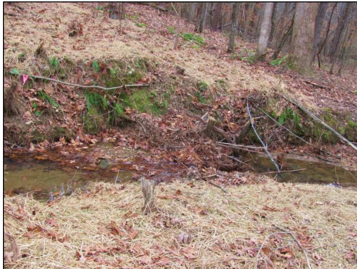
Figure 4. Representative stream crossing approach that was closed with mulch treatment.
