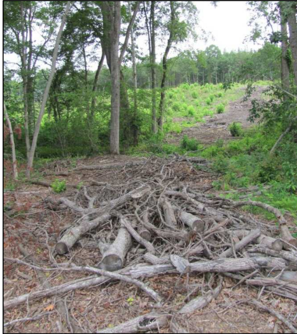
Figure 3. Representative stream crossing approach that was closed with slash treatment.
