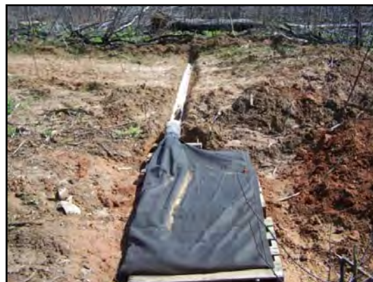
Figure 1. Dirtbags® installed on bladed skid trail.
