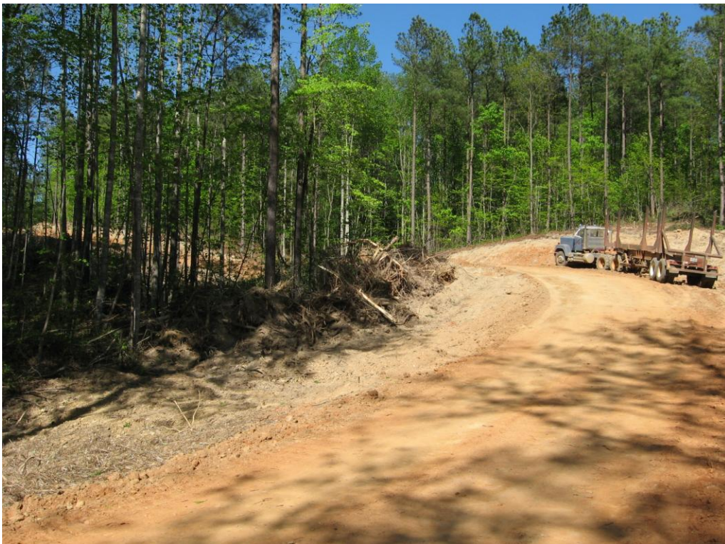
Figure 4. During harvest phase at crossing previously shown in Figure 3.
