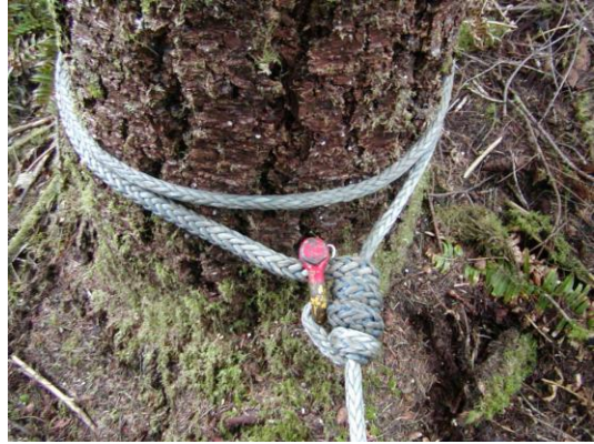
Figure 3. Termination of guyline with shackle
