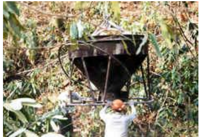
Figure 5: Two chokermen line up the bucket before opening the faucet in order to place the lime.
