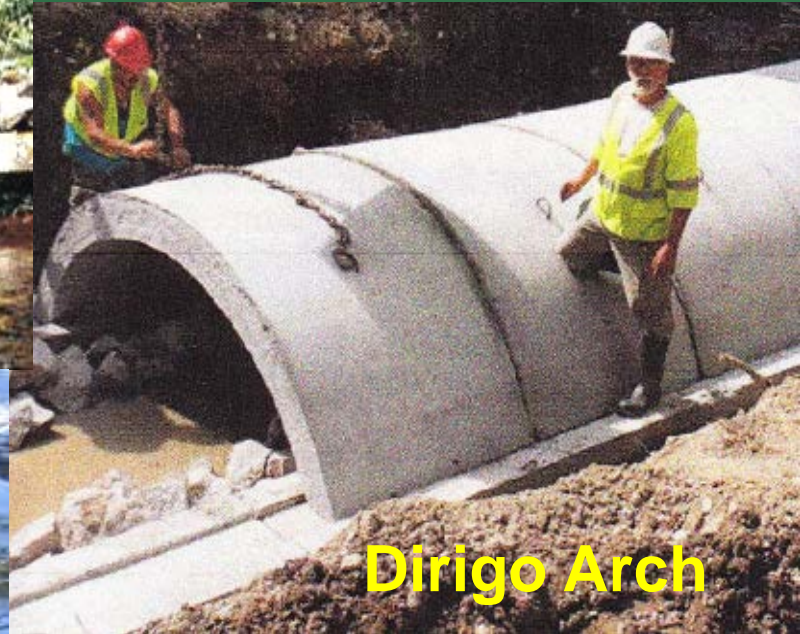
Embedded Culvert
