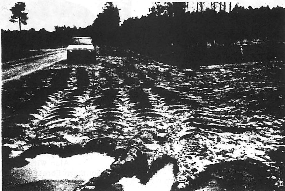
Fig. 1: Mats installed at the intersection of the highway and haul road helped keep mud off the highway.
