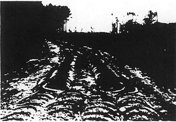
Fig. 4: Mats on haul road to protect site and control mud on tires.
