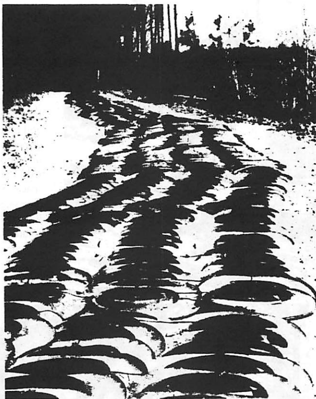
A 600-foot trail of Terra Mat protects a dirt road in Sladesville, N.C. The mats are made from old tires.
