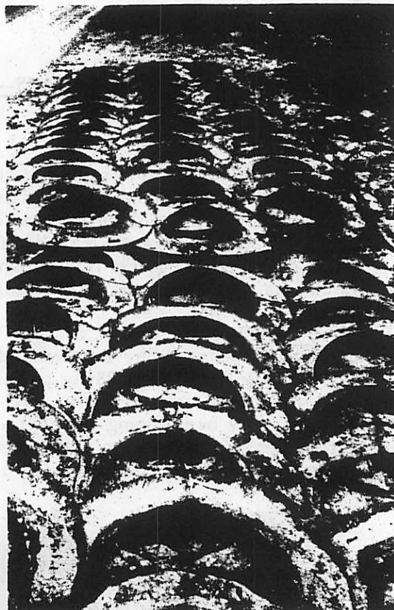
Fig. 3: Mats installed on logging job.
