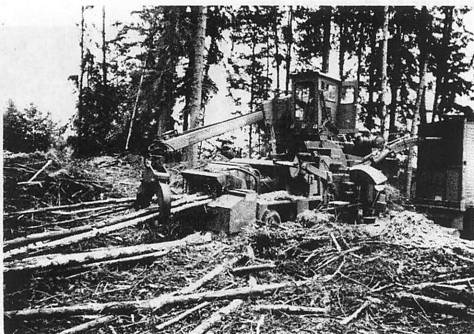
Figure 3. Peterson Pacific Corporation debarker, mounted on a Morbark Model 22 chipper.
