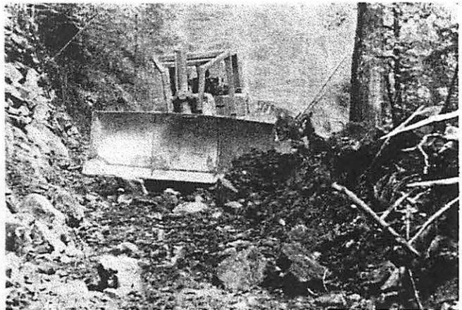
Figure 5.--Typical dozer excavation in the trench.
