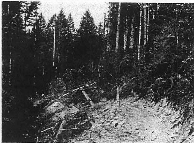
Figure 3.--Begin excavation at the upper slope stakes.
