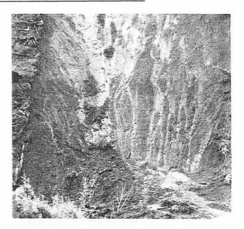
Figure 2.--Combination of translational rotational slide caused by sidecasting and high pore water pressure.
