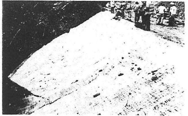
Figure 6.--Slope seeding covered with straw blind.
