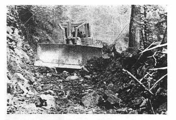
Figure 5.--Typical dozer excavation in the trench.
