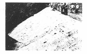
Figure 6 .-- Slope seeding covered with straw blind.
