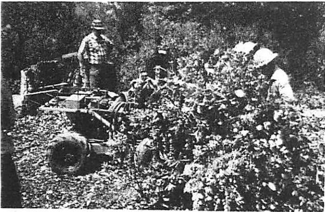
Figure 4. Forestry power module used in brush bundling operation.
