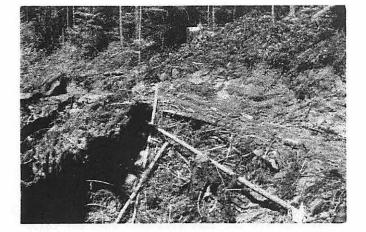
Figure 4.--As excavated material is drifted on logs and other debris, it will form the pioneer road.
