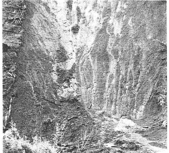
Figure 2.--Combination of translational - rotational slide caused by sidecasting and high pore water pressure.
