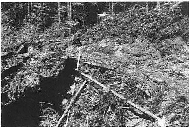
Figure 4.--As excavated material is drifted on logs and other debris, it will form the pioneer road.
