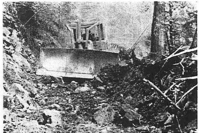
Figure 5.--Typical dozer excavation in the trench.
