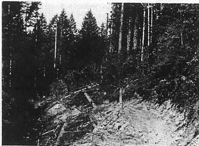
Figure 3.--Begin excavation at the upper slope stakes.
